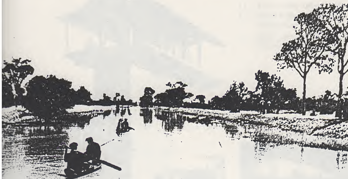
Newly built canal « April 17 » of 49 kilometers long in the North-east region, irrigating tens thousands of hectares of lands.
