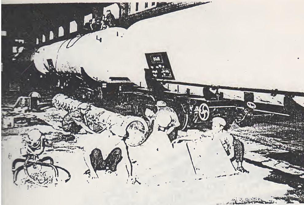
Construction of tank - waggons
