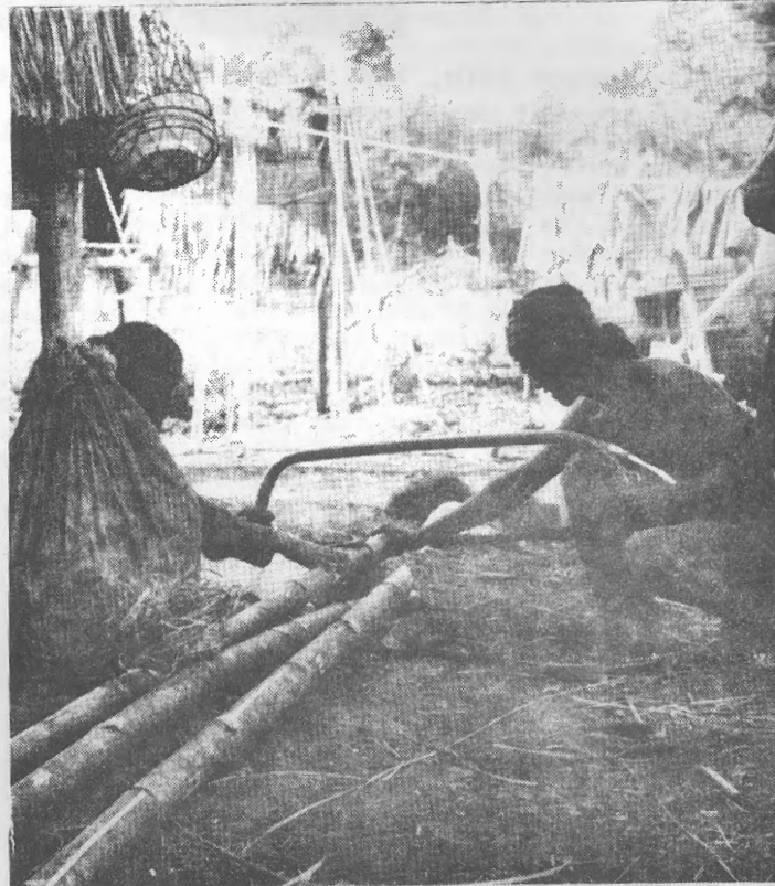
Work goes on in the villages - here bamboo is sawn for house building
